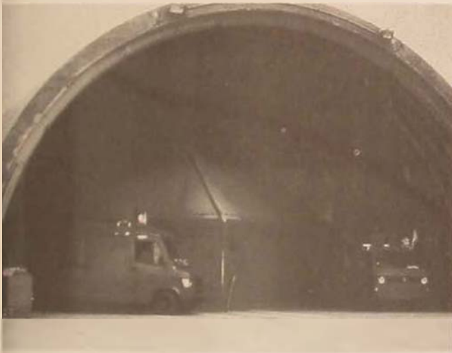
Concrete and earth provide necessary protection for people and equipment at today's theater air base.
